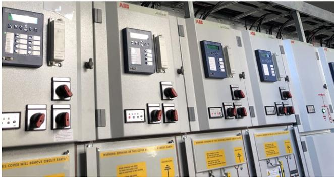
In late 2017 PBA commenced a yearlong project upgrading the 11kV reticulation system at Ravensdown's Christchurch Fertiliser Plant. As a continuous manufacturing operation utilising co-generation units this project utilised the full skill set of the PBA team headed by Tom Wech and Hayden Burrows to maintain operation of the plant as the various upgrades were applied. In addition to the initial programmed works the PBA team were able to identify
